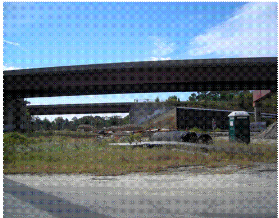
Bridge on I-164 at the Coast Guard Blvd. in the City of Portsmouth.
